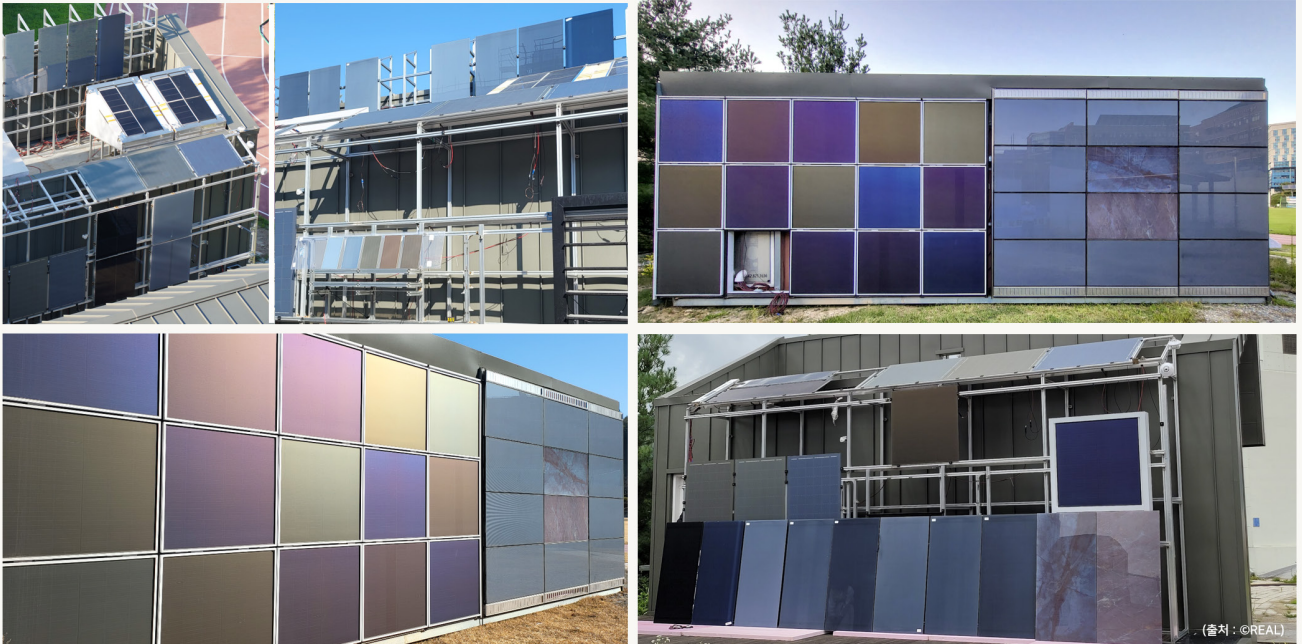
(BIPV Field Test Facility @REAL, 한밭대학교)
